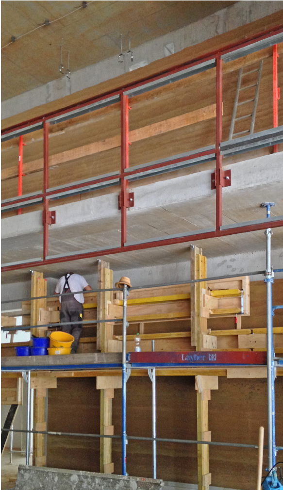
07-09 The construction process showing the travelling formwork principle
