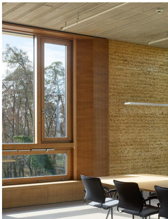
09 Acoustic timber window surrounds
