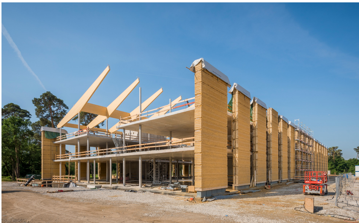
12 The building shell with the assembled prefabricated rammed earth sections
