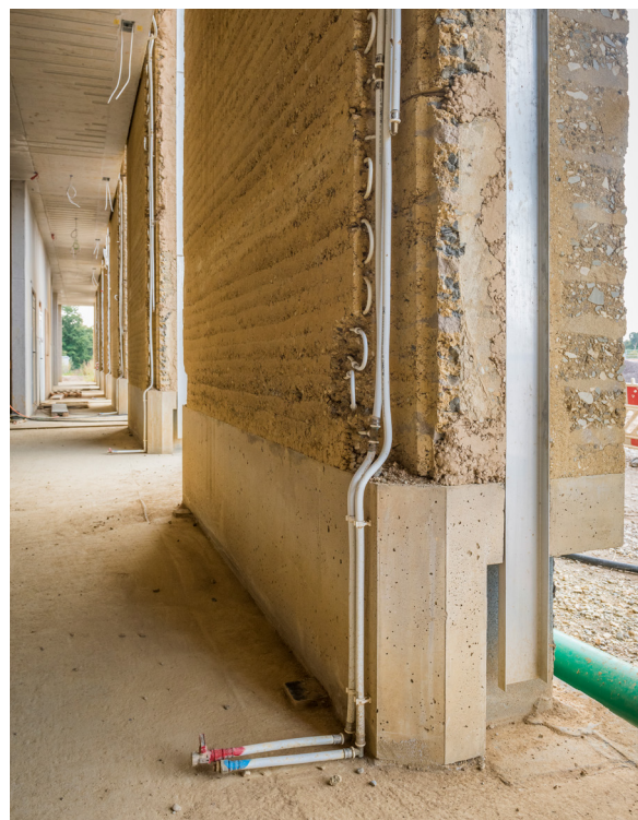
11 Inner face of the rammed earth elements with integral wall heating, core insulation and window rebate
