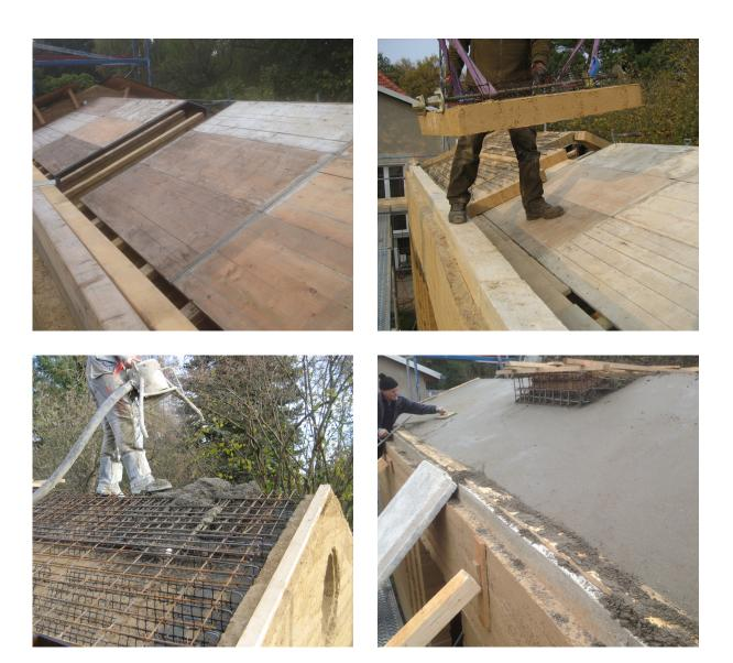
The gable walls had to end in an incline corresponding to the pitch of the roof so that the wall crown can bear the load of the massive earth panels. And this was the next lessen we learned.
