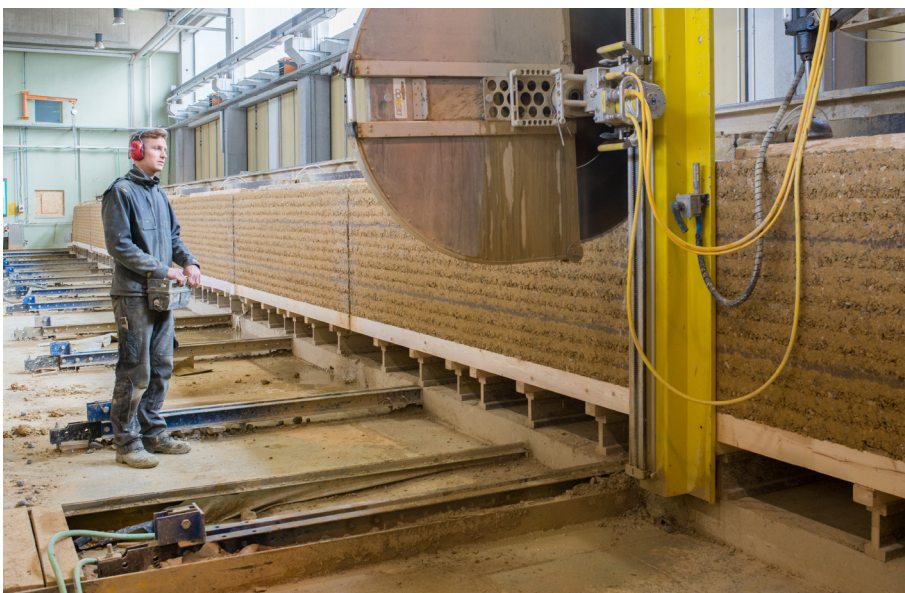
05 Cutting the prefabricated rammed earth wall into sections
