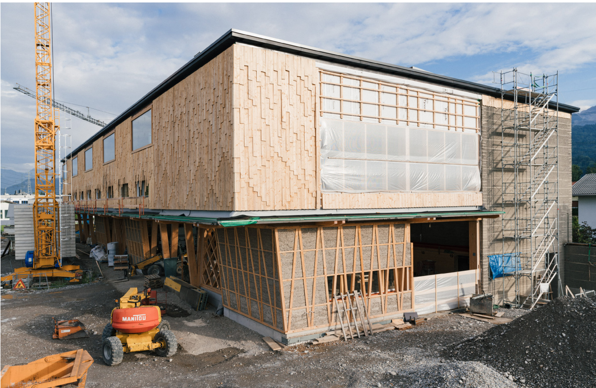
11 The building is a hybrid rammed earth/solid wood construction
