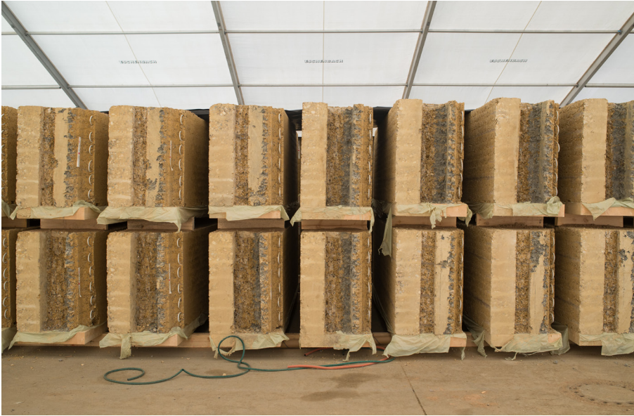
06 Drying the prefabricated rammed earth elements
