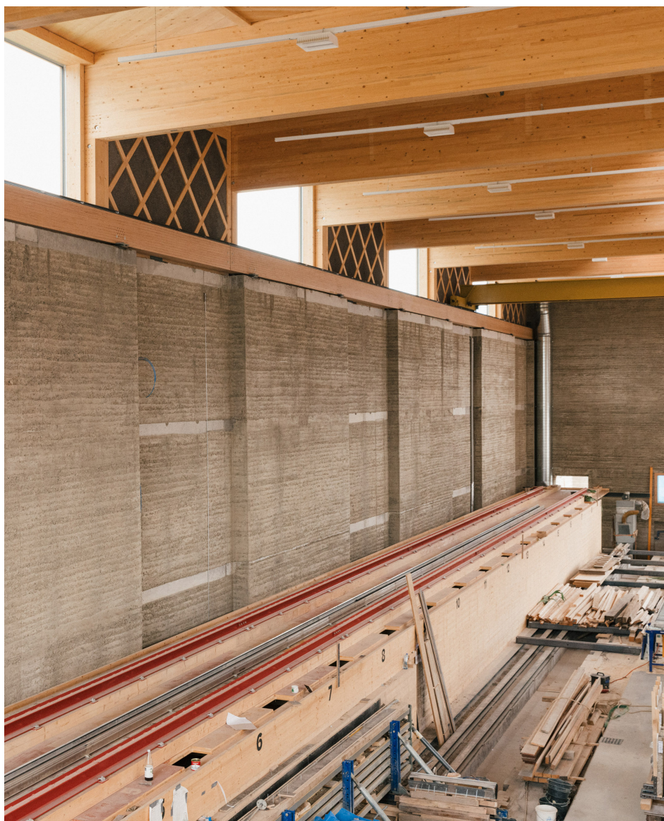
09 The solid timber roof rests on the loadbearing rammed earth walls
