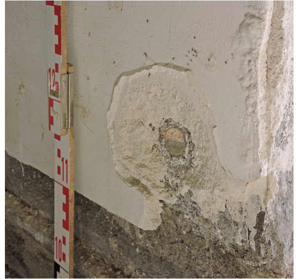
09a and b The injection holes for the 1980s chemical horizontal damp proofing barrier are too far apart. In addition, the injection agent was chemically and physically incompatible with the stone it was injected into.
