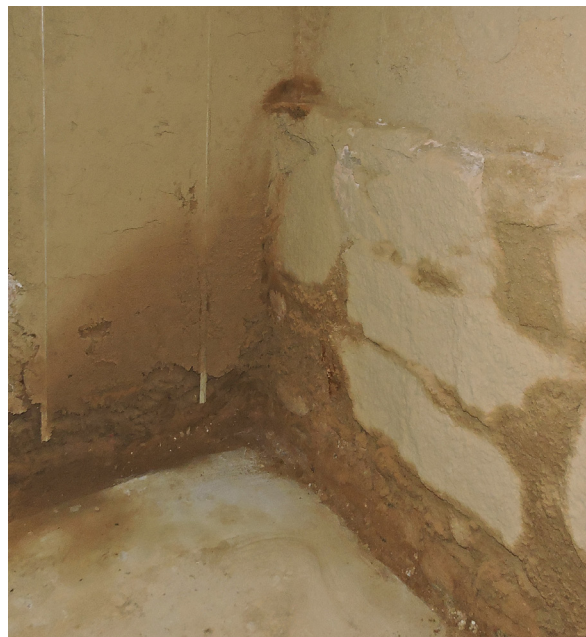
08b Sacrificial plaster with clearly recognisable localised incidence of hygroscopically increased moisture
