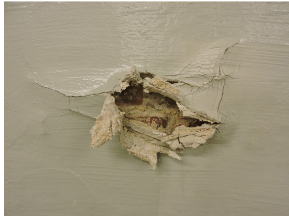
03a and b The "restoration" of a basement using barrier plaster without installation of a horizontal barrier. 5 years on, the evaporation zone has shifted upwards and the coating has burst open.
