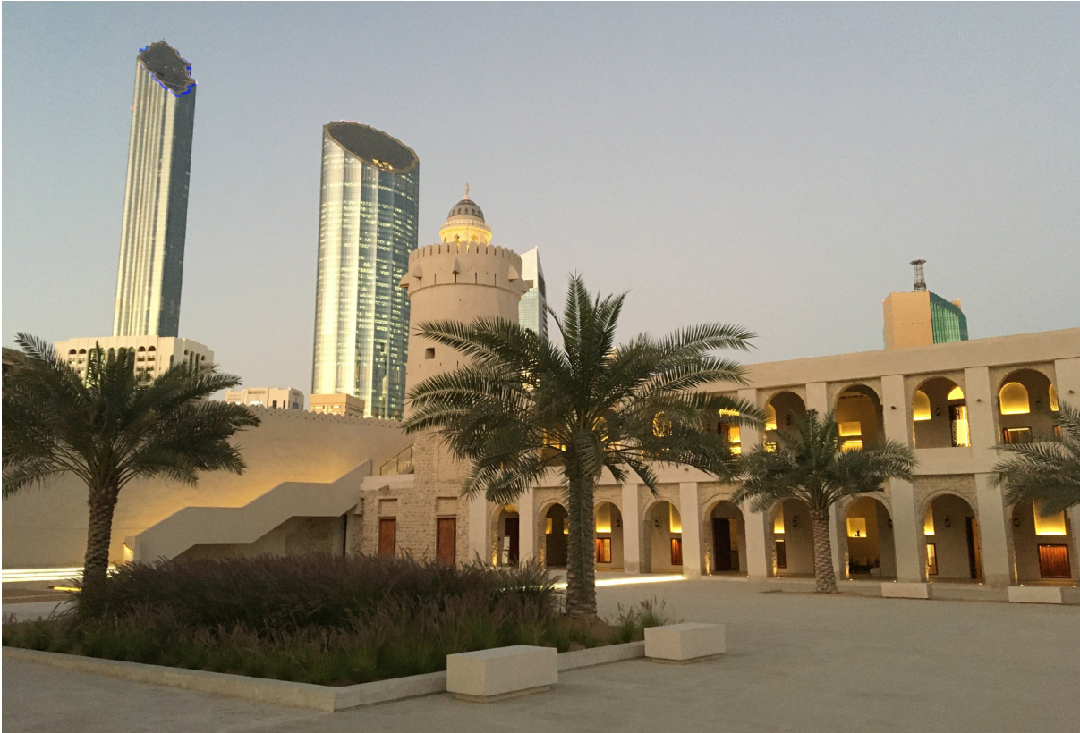
10b Qasr al Hosn, Abu Dhabi, UAE, after completion of desalination works
