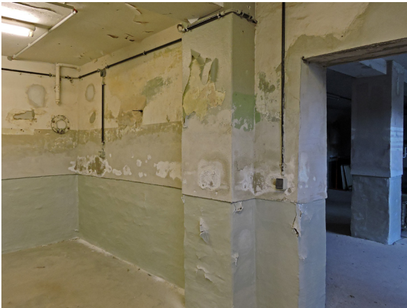
03a and b The "restoration" of a basement using barrier plaster without installation of a horizontal barrier. 5 years on, the evaporation zone has shifted upwards and the coating has burst open.
