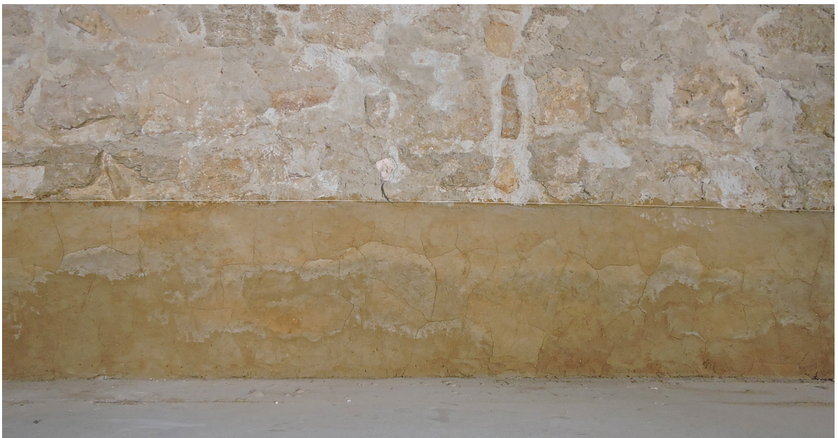
10a Clearly visible indications of desalination during the third cycle of desalination measures
