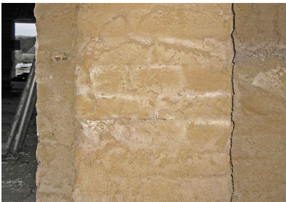
06a and b Salt penetration into the sacrificial plaster can be seen as whitish salt deposits on the surface or dark areas that do not dry out. Depending on the type and combination of materials in the existing structure, the salt concentration may be higher in the masonry mortar (left) or in the bricks (right).
