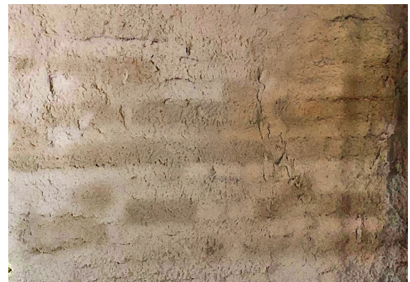
06a and b Salt penetration into the sacrificial plaster can be seen as whitish salt deposits on the surface or dark areas that do not dry out. Depending on the type and combination of materials in the existing structure, the salt concentration may be higher in the masonry mortar (left) or in the bricks (right).
