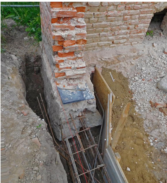
08a Installation of the horizontal damp proofing and local foundation reinforcements
