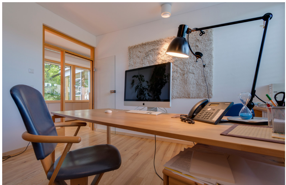
04 Earth building board walls, softwood fibreboard ceilings, clay plaster and lime paint
