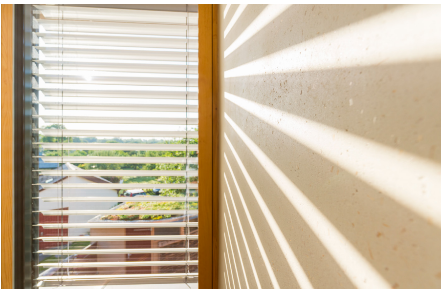
08 Clay finishing plaster with straw additive visible in the surface structure
