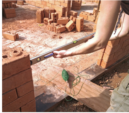
09–11 Uneven brick courses must be corrected using sand, especially at the base of the wall as irregularities affect the subsequent brick courses. Irregularities in vertical perpendicularity can be corrected with the help of a rubber mallet.
