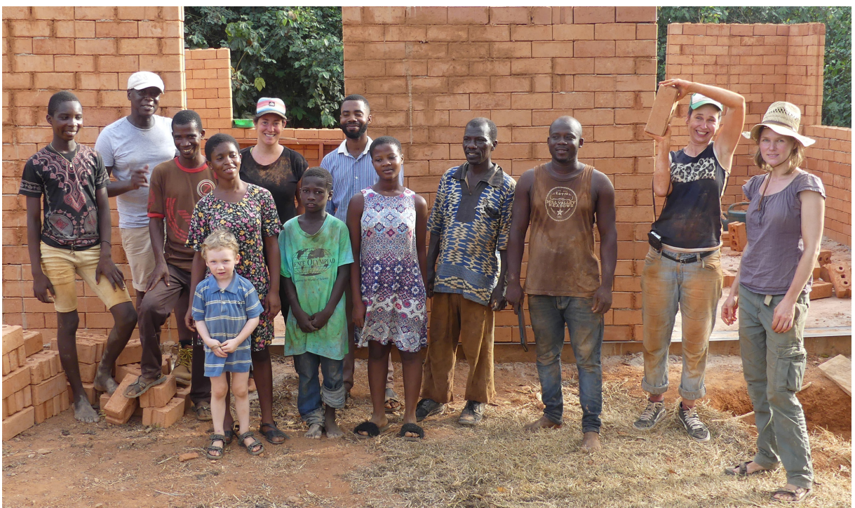
23 Africa meets Europe: Knowledge transfer, exchanging ideas, gaining insight. Some members of the construction team in front of the stacked walls of the first experimental laterite LEGO building
