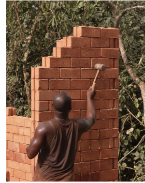
09–11 Uneven brick courses must be corrected using sand, especially at the base of the wall as irregularities affect the subsequent brick courses. Irregularities in vertical perpendicularity can be corrected with the help of a rubber mallet.
