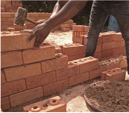
09–11 Uneven brick courses must be corrected using sand, especially at the base of the wall as irregularities affect the subsequent brick courses. Irregularities in vertical perpendicularity can be corrected with the help of a rubber mallet.
