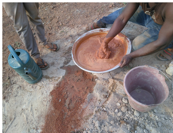
12+13 Experimenting with the recipe of the grouting mixture for pouring into the vertical holes of the laterite bricks
