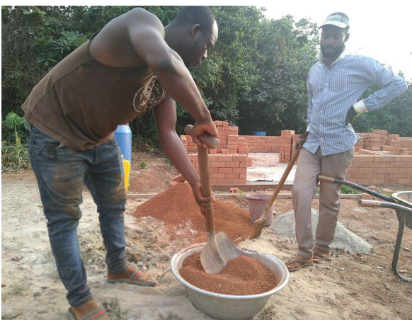
12+13 Experimenting with the recipe of the grouting mixture for pouring into the vertical holes of the laterite bricks
