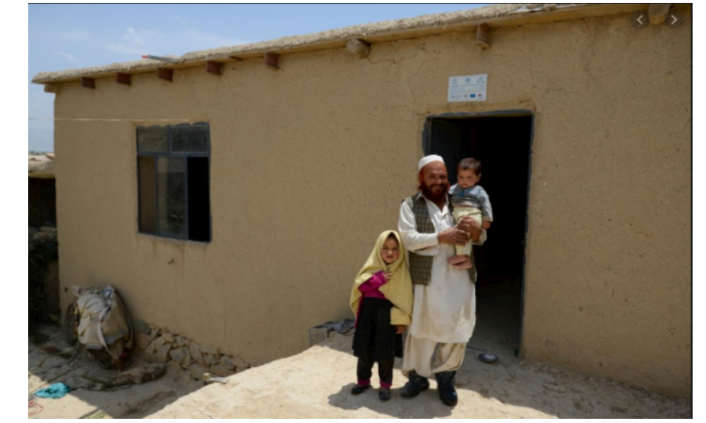
PIC 3. Adobe house with stone foundation and soil-straw plaster ,
